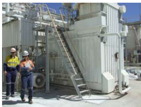
Assessment of Steam Boilers at Kwinana Pigment Plant
