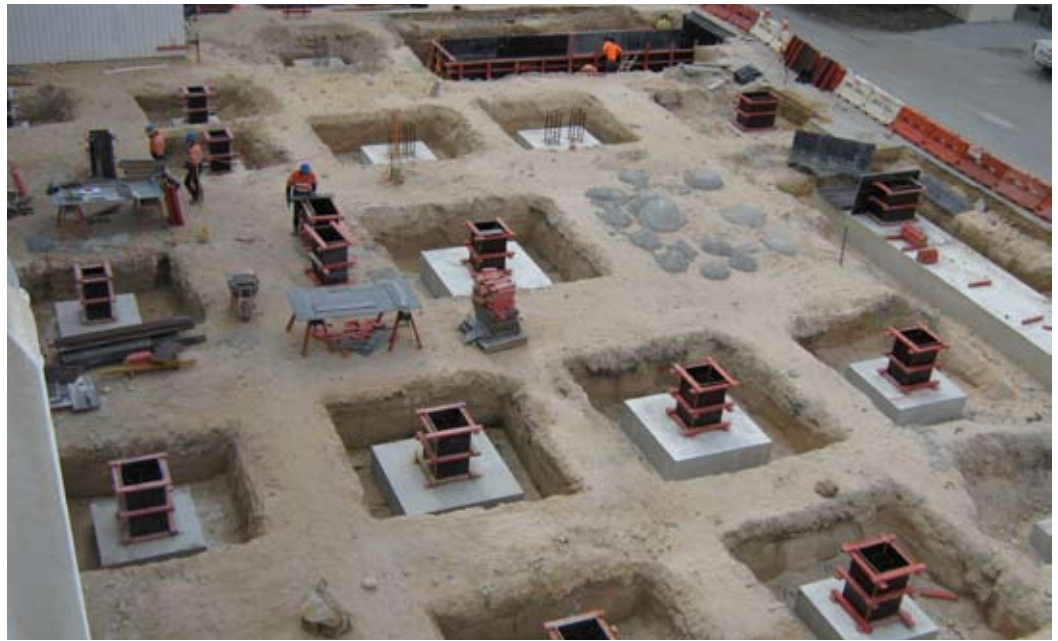
Expansion works underway at Kwinana
